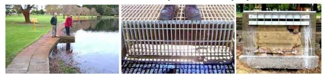
**Above left,** the outlet drain enclosure juts out from the lake edge. **Middle**, it consists of a weir protected by a grille to prevent leaves entering. **Right,** new grille early 2011, previous calculations no longer apply.
