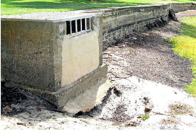
The same record rainfall leads to a flow reversal into the lake through what should have been the outlet , scouring away the sand below and leaving packed leaves and twigs behind the outlet grille..
