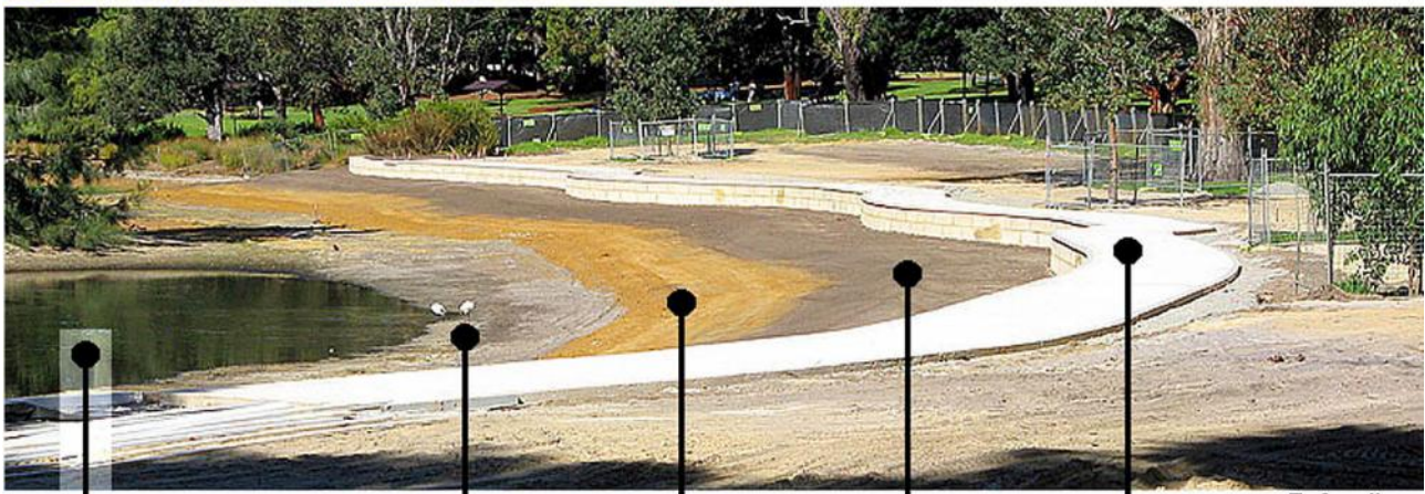
Water Original lake bed Clay layer Soil layer New path 5 April 2018
