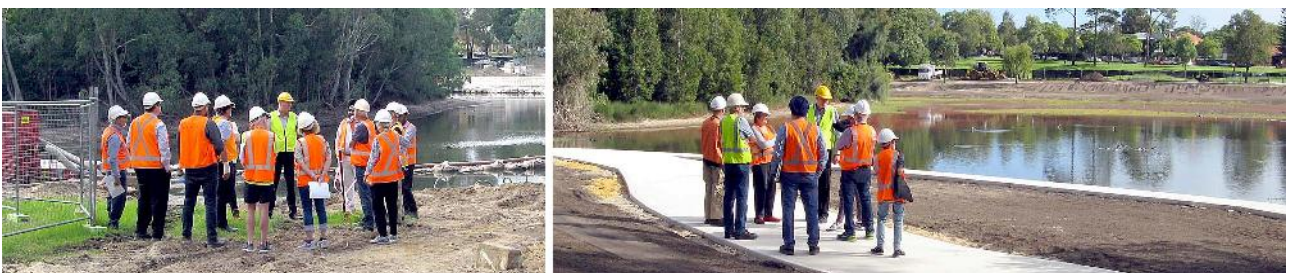
Subiaco staff give Save Our Jewel the opportunity to view progress and ask questions. In yellow facing camera is Gray Stead, Director of Technical Services. Left 6 February. Right 10 April, where across the lake the sloping banks are covered by cloth mesh to prevent erosion until established.
