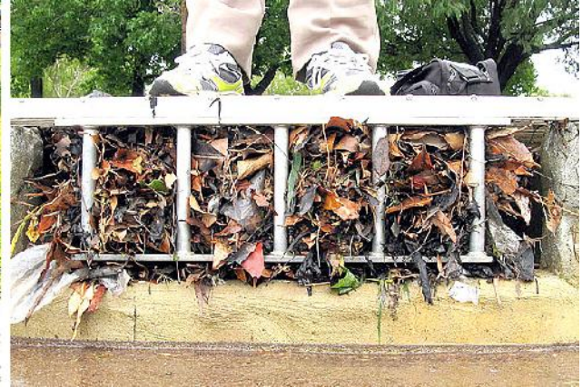
The same record rainfall leads to a flow reversal into the lake through what should have been the outlet , scouring away the sand below and leaving packed leaves and twigs behind the outlet grille..
