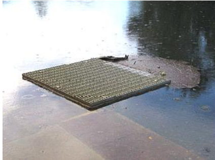
Left two: In May 2014 Water Corporation installed a new grille to the outlet. Unlike the previous grille it offered minimum resistance to the flow and (bottom picture) allowed smooth streamlines over the weir crest. Above two: For those up close on 22 July (when the previous flood picture was taken), the noise of water over the weir threatened to rival Niagara. Five weeks later the lake level was even higher, see next.
