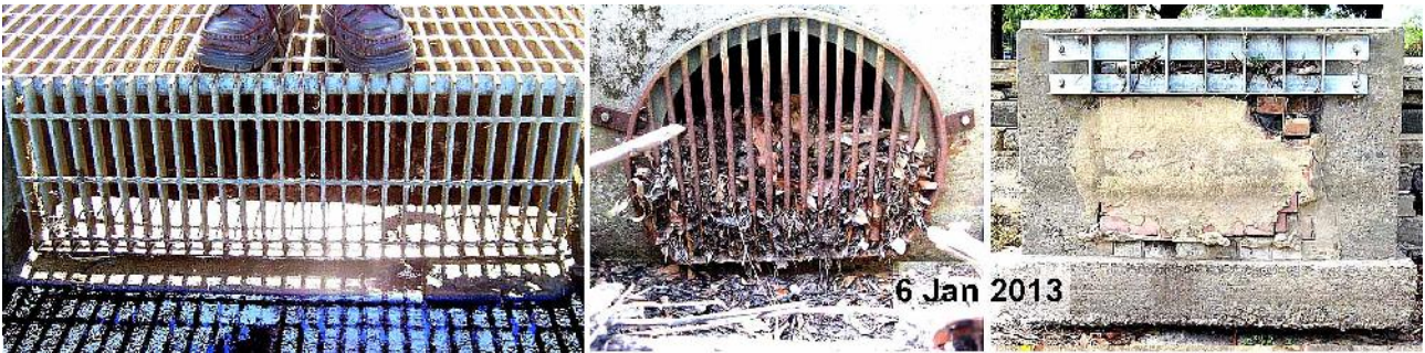
Left: original open grille in 2008. Right: temporary restrictive grille installed early in 2011. The broken brickwork at the right of the weir will be repaired. Middle: start of the outlet pipe running from behind the grille to the ocean. Not easily visible to the eye but here photographed through the grille. How did all that debris get behind the bars? Shouldn't it be in front of the bars? The WC have advised us they will investigate. Below: a new less-restrictive grille was installed in May 2014. The original open grille over the top was retained. The internal bars shown in the middle picture above were removed to allow water to flow more freely, albeit with the disadvantage that the entry of debris would not be prevented.
