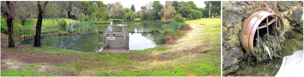
Above left: Kilgor Park Lake after excavations were finished. Right: leaves and weeds pumped to Jualbup
